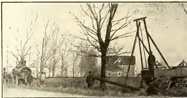
RAISING POLES BY MEANS OF GALLOWES ATTACHED TO OLD EMERGENCY WAGON
